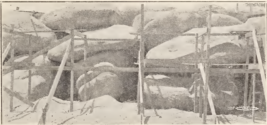
4. Showing outside coat of cement. Applied with cement guns to a thickness varying from 2 to 5 inches.
